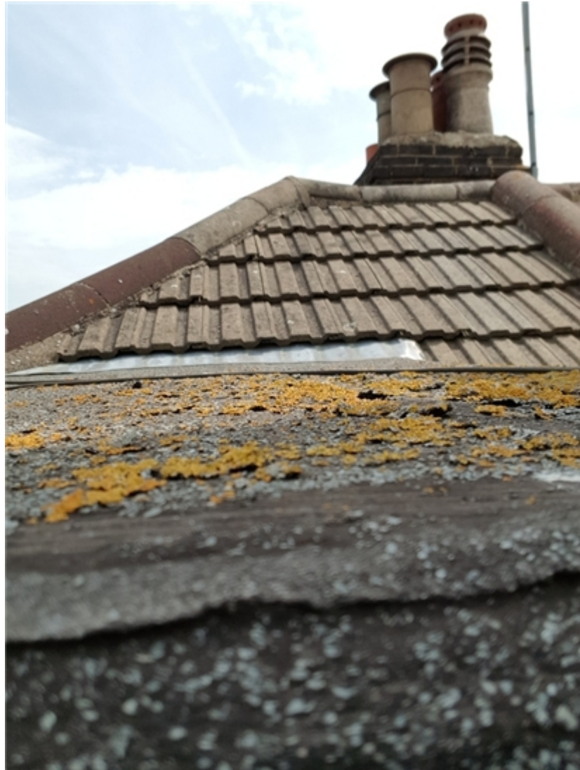
Limited flat roof covering inspection.
