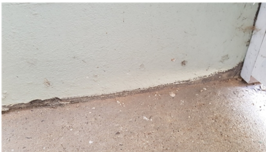
Chemical injection damp proof course.
