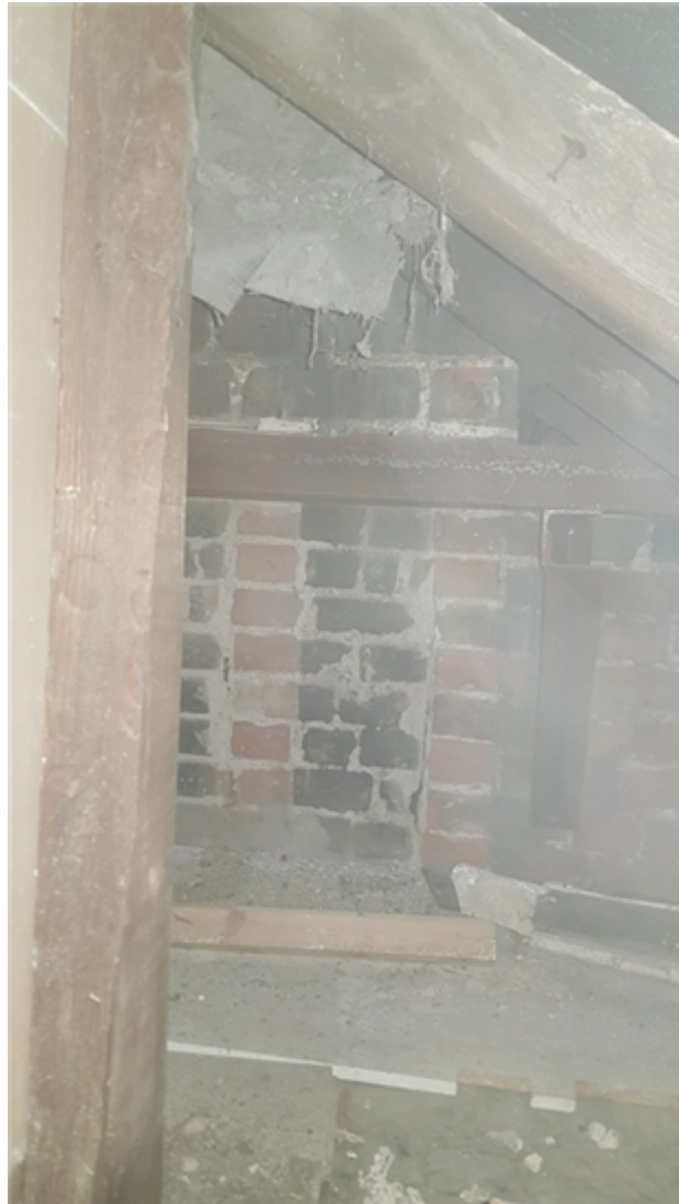
Support for rear chimney.
