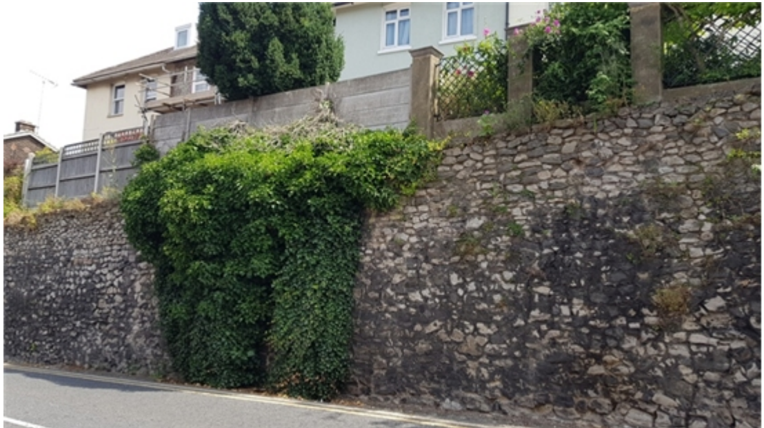
Rear retaining wall.
